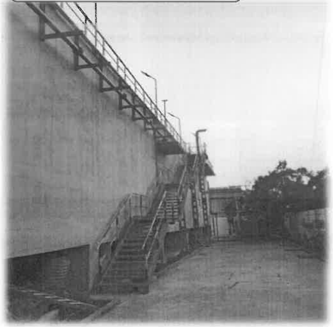
Above ground level effluent Plant
